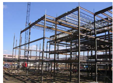
Figure 2 - Steel erection underway
